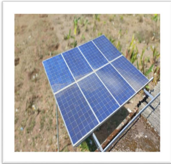
1.5 KW x 3 KV solar off grid power system installed at SN College Chathannur.
