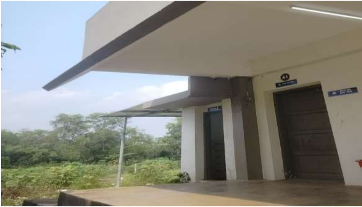
CCTV ON ARTS BLOCK ENTRANCE
