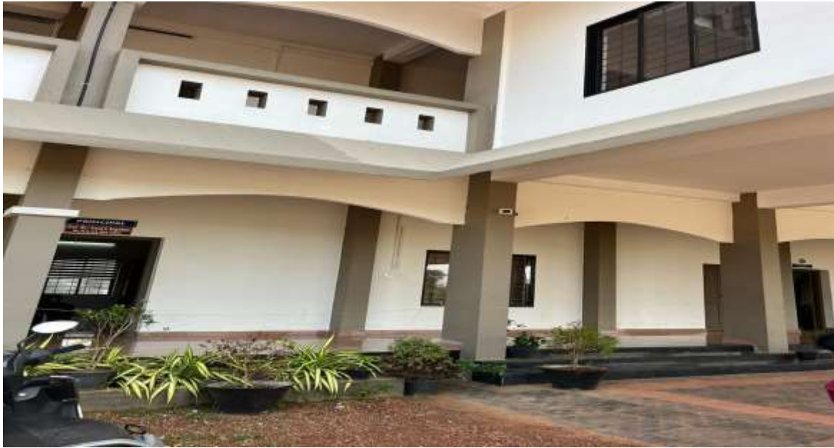
CCTV ON MAIN BUILDING ENTRANCE
