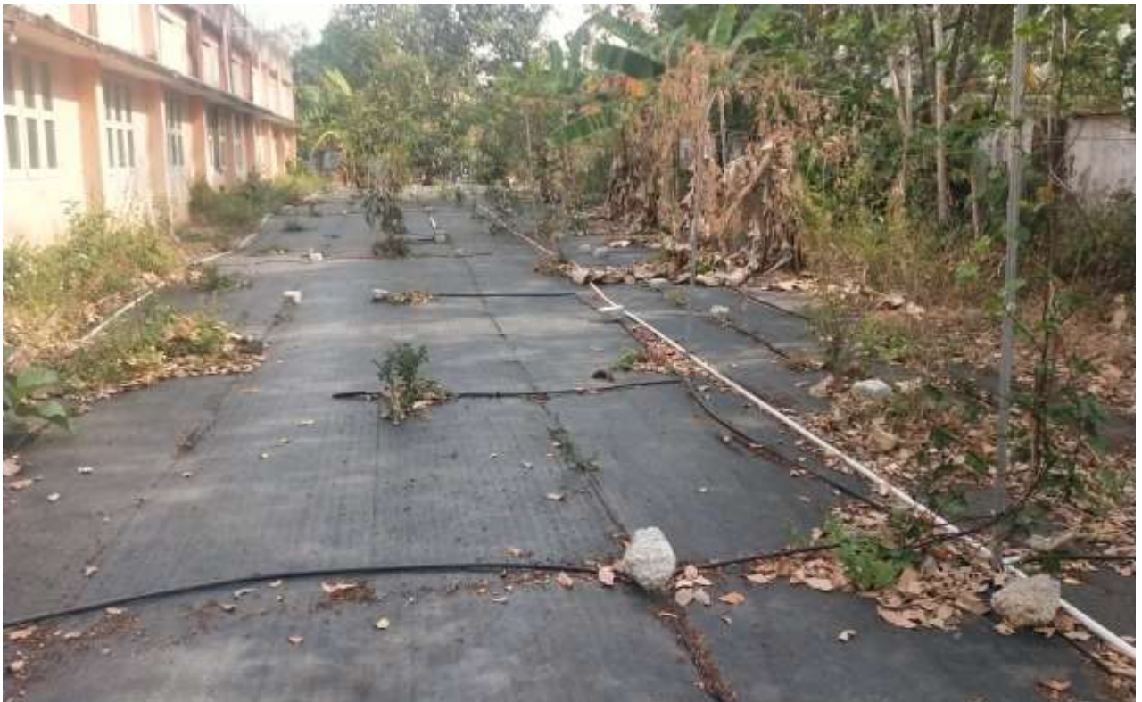
Waste Water Recycling
